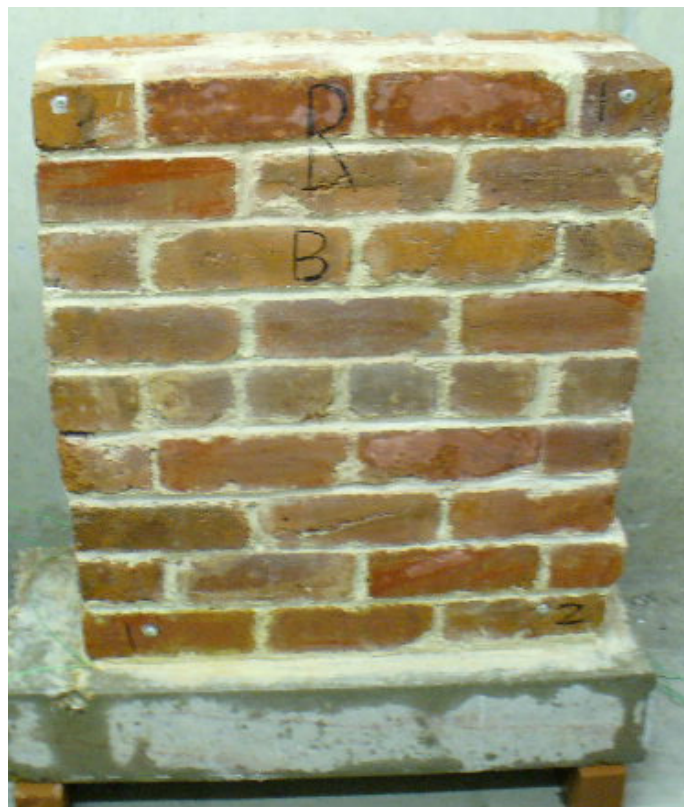
Figure 12: Wall panel R view after drying process - no visible damage
