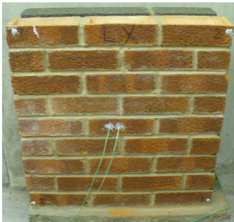
Figure 10: Wall panel LX view after drying process - no visible damage
